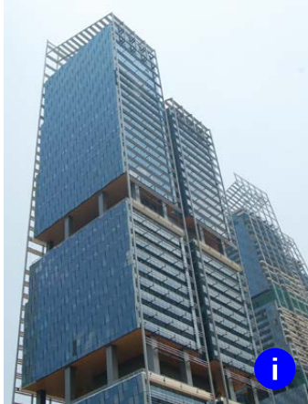
South Beach Tower
